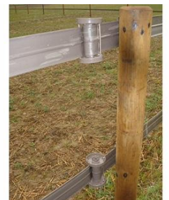
Place tension part and re-insert locking plate
